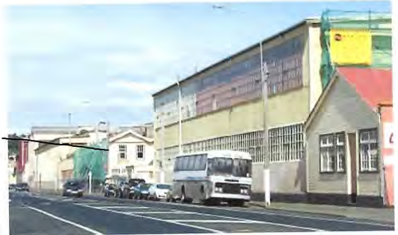
The Hillside Workshops stretch for over 500 metres along Hillside Road, South Dunedin.
