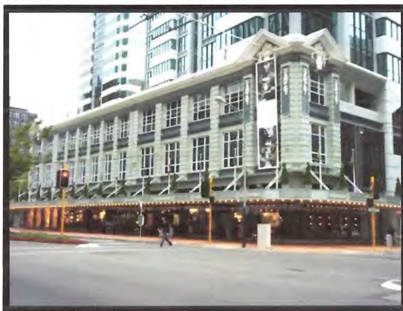
Kirkcaldie and Stains Department Store Façade. Photographed by Rachel Connolly 10/01/2009. Copyright NZ Historic Places Trust
